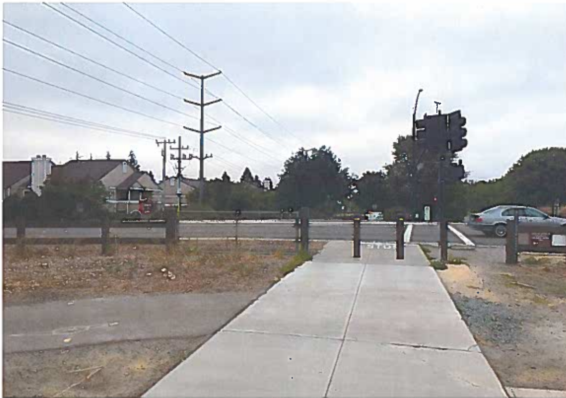
Photo 1: Existing Iron Horse Trail Crossing at Bollinger Canyon Road, Looking South
